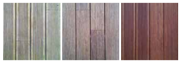
weathered, dirty decking weathered, cleaned decking refinished decking
