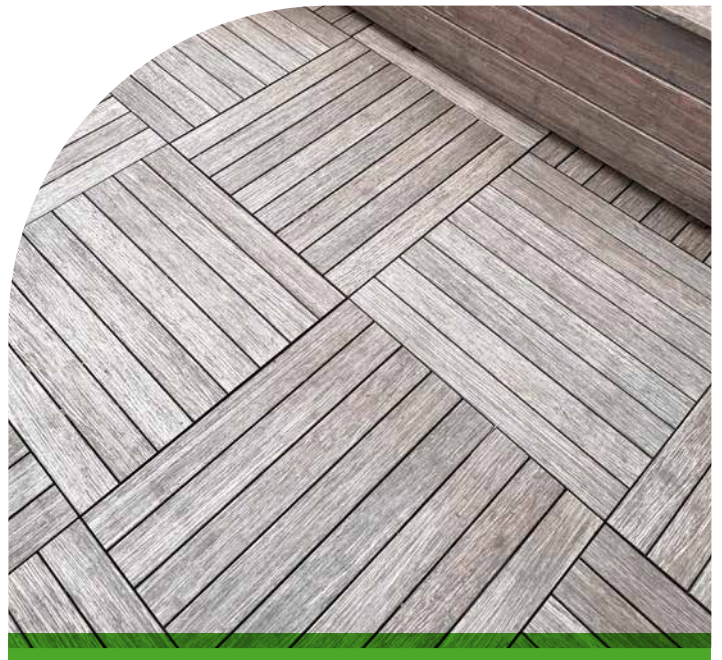
Bamboo balcony Deck tiles aged 12 months in full sun on rooftop application - Philadelphia, United States of America
